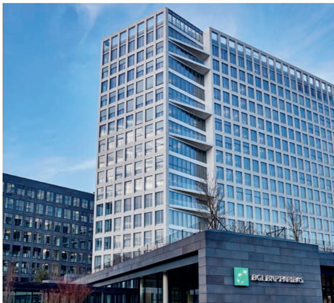
BGL BNP Paribas, Luxembourg, Luxembourg ClimaGuard® Dry | Double skin facade, anti-condensation coating on exterior surface Architect: M3 Architectes | Photo: © Frank Weber
