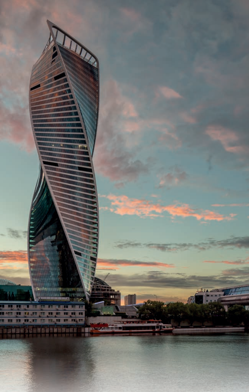
Evolution Tower, Moscow, Russian Federation SunGuard® HP Neutral 60/40 | "Twisted" facade with cold bent insulating glass Architect: Tony Kettle | Photo: © Olga Alexeyenko
