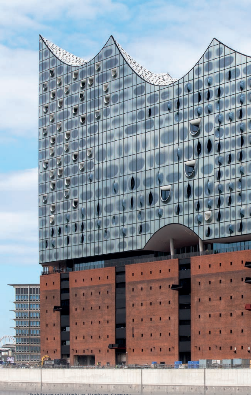
Elbphilharmonie Hamburg, Hamburg, Germany SunGuard® HD Light Blue 52 | 3-dimensional gravity curved, ceramically printed, laminated insulating glass Architect: Herzog & De Meuron, Basel | Photo: © Cordelia Ewerth
