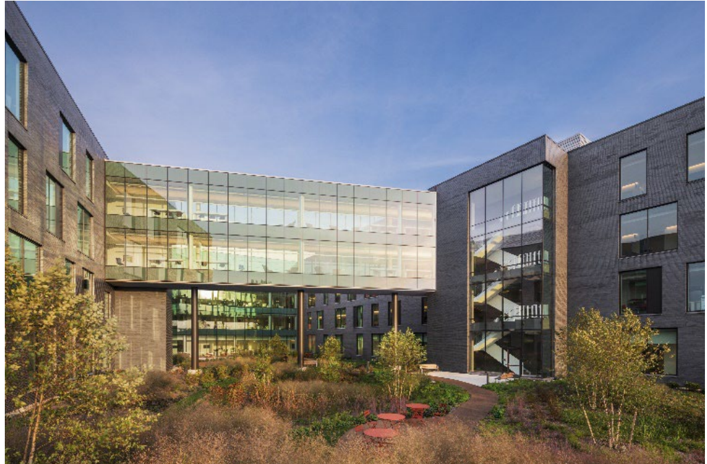
Figure 1 – Sputter Coated Glass Installed at Penn Medicine at Radnor Medical Office Building.
